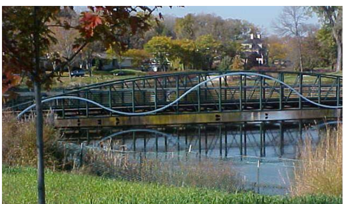
Walking bridge over Calhoun Pond, one of the many projects involved in the Chain of Lakes partnership
