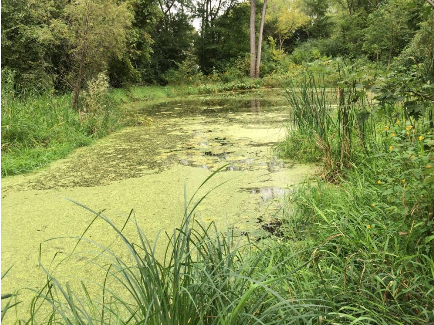
Q:\Departments\O&M\Annual Inspections\2015 Inspections\Gleason Ponds (Image 7345)
