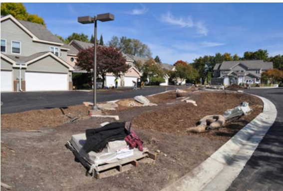
Three raingardens under construction at Parkway Place Townhomes
