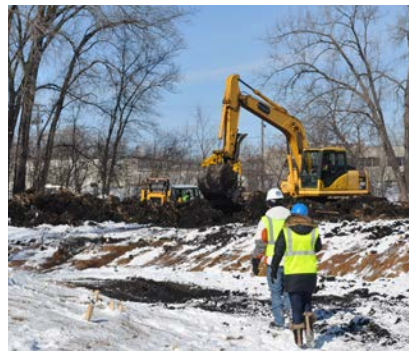
Permitting staff inspecting a construction site
