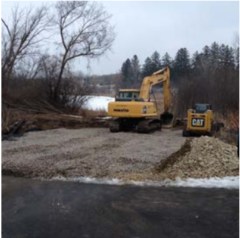
Construction work at Long Lake Creek
