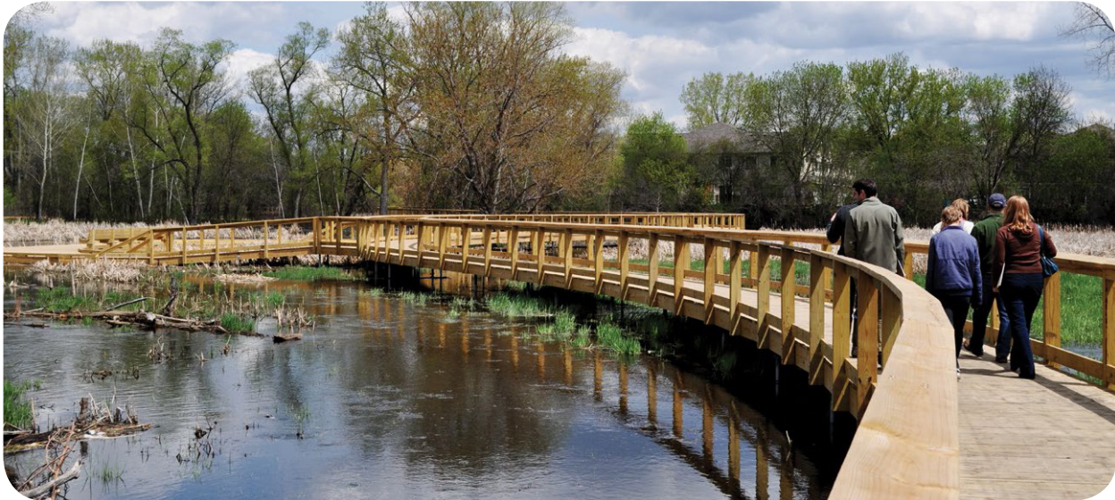
Boardwalk system under construction along Minnehaha Creek
