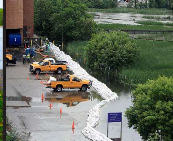
Methodist Hospital staff using sandbags to fend off high water (credit: Jeffrey Thompson/MPR News)
