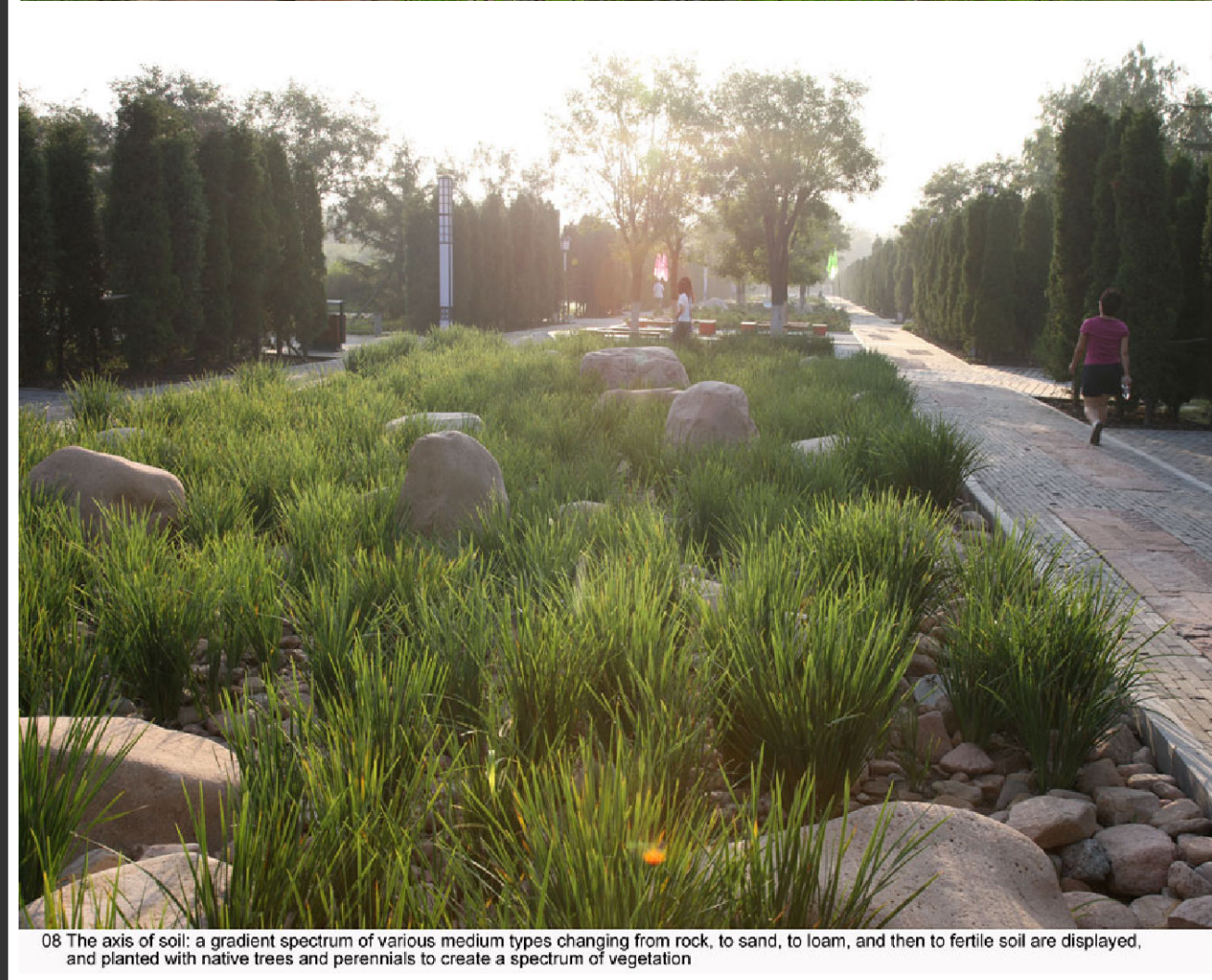
Bioretention/ Biofiltration Swales
