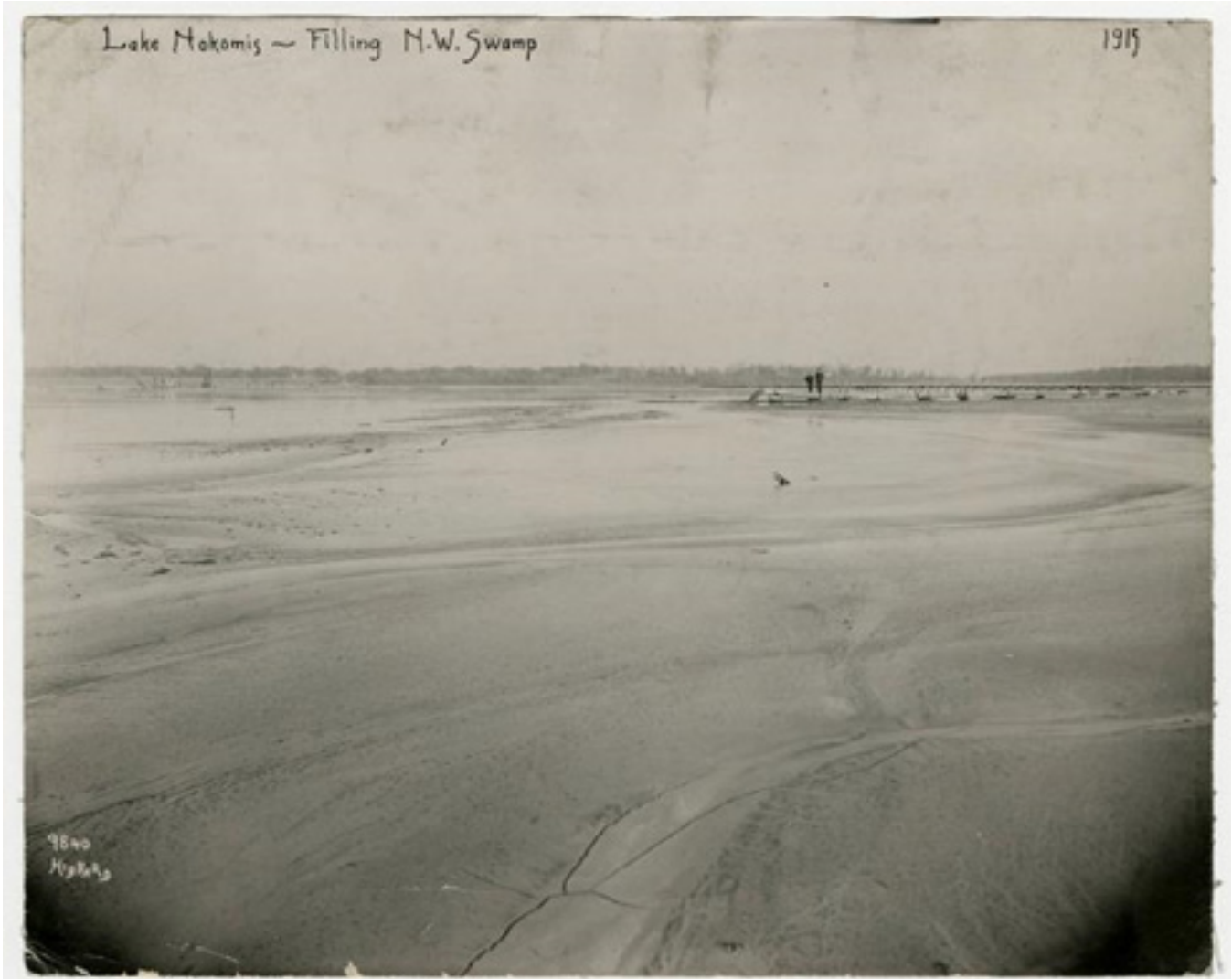
Figure 30: Filling Swamps. Dredge fills were placed over a swamp northwest of Lake Nokomis in 1915. (Credit: MPRB, 2021)
