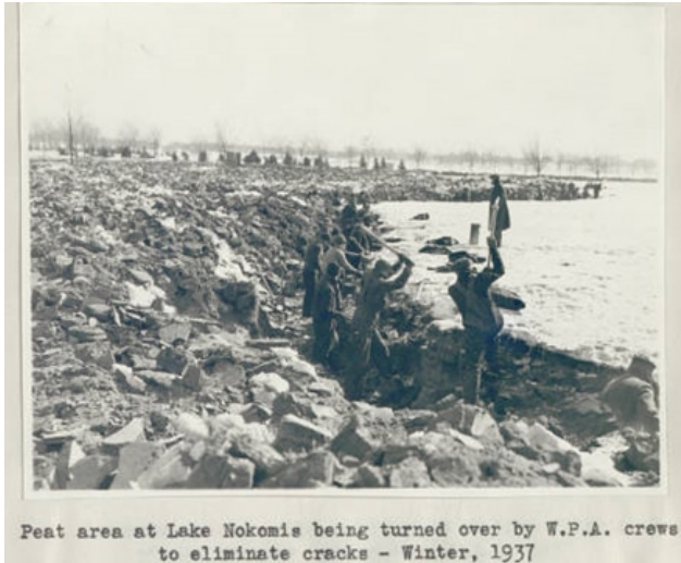
Figure 39: Overturning Peat. Peat soils at Lake Nokomis being turned over by WPA crews to eliminate cracks (Source: Minneapolis Board of Park Commissioners, 1937)
