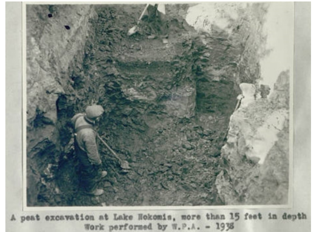
Figure 40: Peat Excavation. WPA crews excavating peat that was more than 15 feet in depth (Source: Minneapolis Board of Park Commissioners, 1938)
