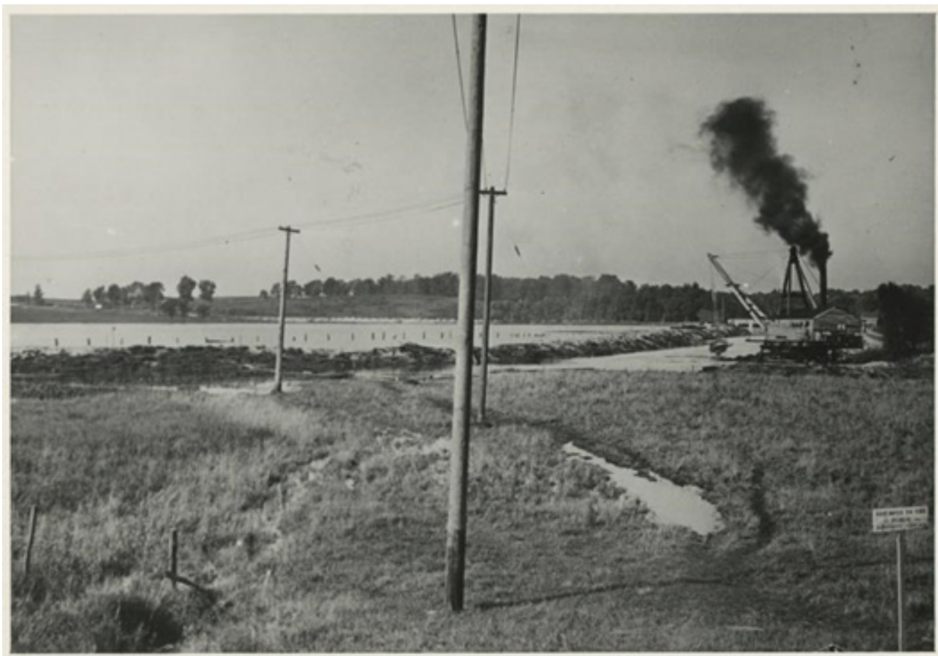
Figure 29: Dredge at Lake Nokomis. Dragline dredge removing wetland and lake soils in 1914. (Credit: Wirth, 1945)
