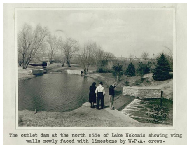
Figure 77: Lake Nokomis Outlet. Photo Caption: The outlet dam at the north side of Lake Nokomis showing wing walls newly faced with limestone by W.P.A. crews. (Credit: Minneapolis Board of Park Commissioners, 1939)
