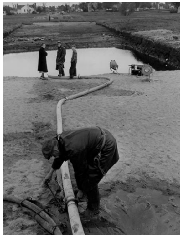
Figure 37: Street Excavation. Pumping out water from a street excavation on 15th Avenue South near 58th Street on May 13, 1941. (Credit: Hennepin County Library, 2021a)
