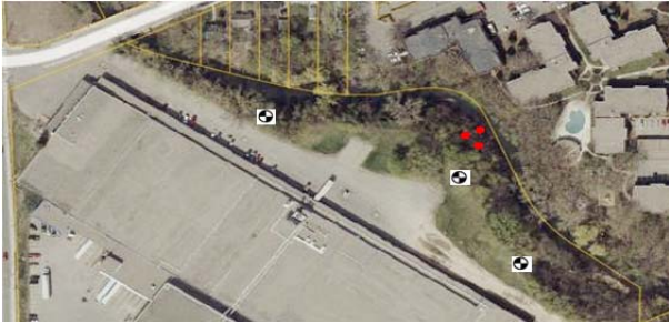
Figure A.8. Approximate locations of piezometer installations (solid red circles) within wooded riparian area of creek and soil borings completed with a drill rig (black and white circles) in the upslope lawn area.
