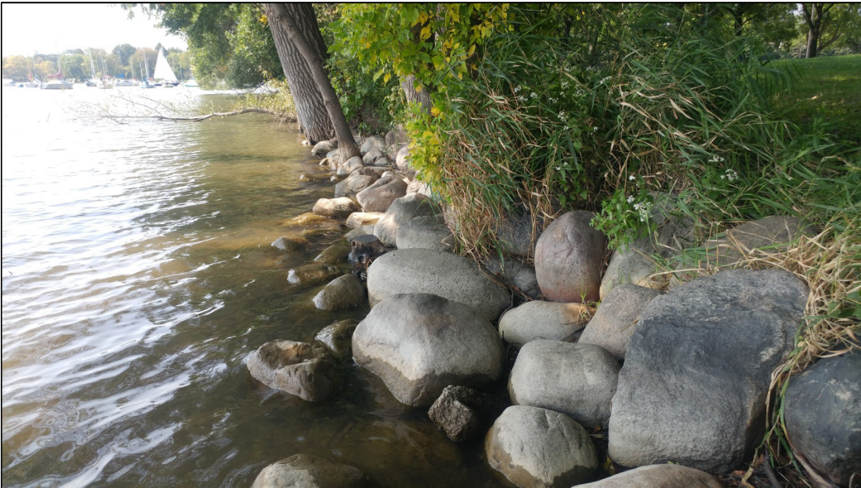
Photo 11. Existing Conditions – Riprap/boulders stabilizing west shoreline.
