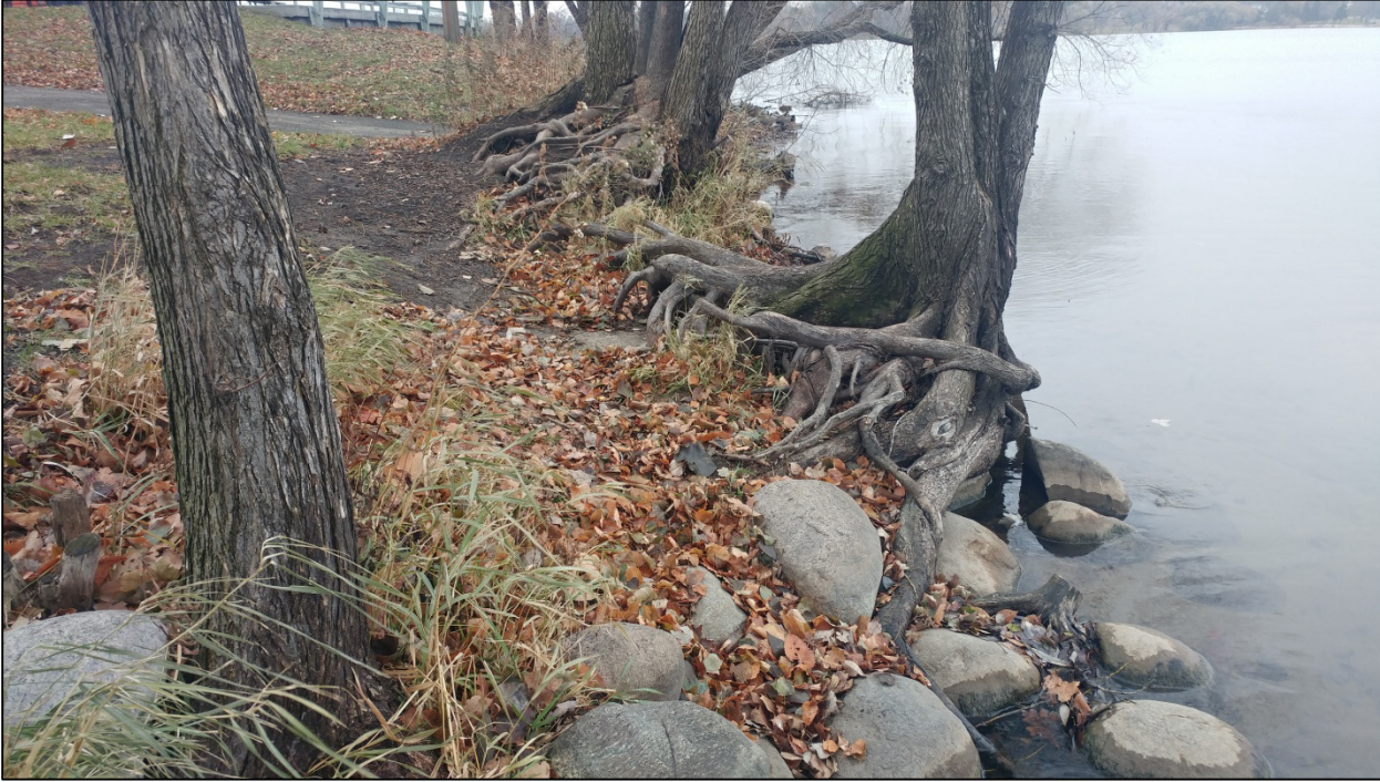
Photo 6. Existing Conditions – Erosion along lake’s west shoreline (south of west beach).
