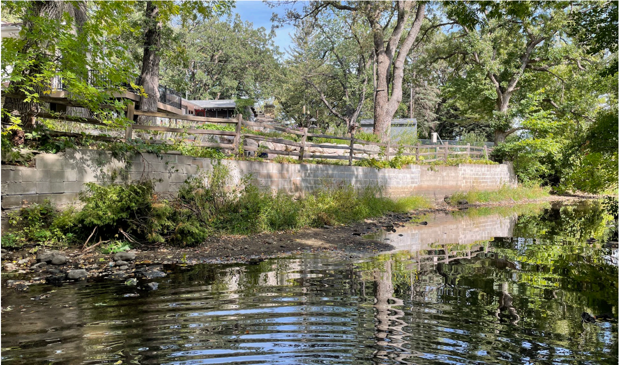
Figure 3: Cinderblock wall downstream of utility crossing.
