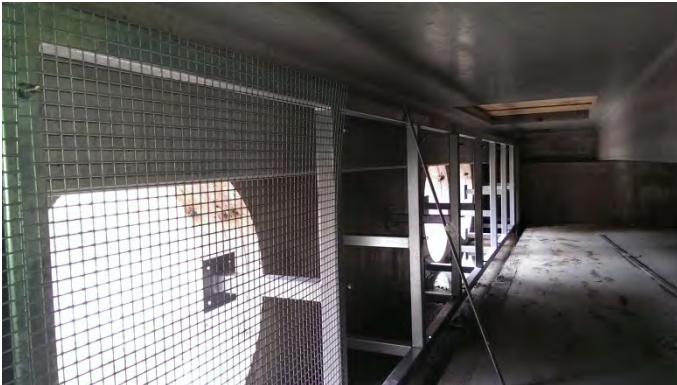
Structural framing and steel backer screen construction for curtain wall pre-treatment system. When complete, a sacrificial filter fabric will be mounted against the backer screen to filter fine particles from entering the three 48-inch openings to the infiltration system. A large vault opening indicated in upper right (background) of photo allows maintenance access for periodic removal and replacement of fabric.
