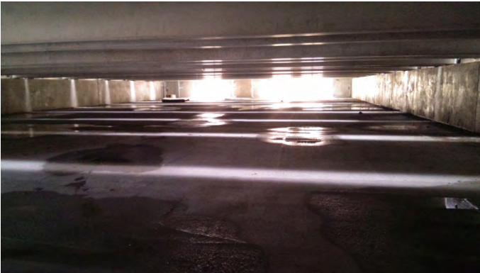
Looking north inside Engel Street detention vault during construction. Large sun-filled openings are for eventual connection with 48-inch perforated pipe network of adjacent infiltration basin.
