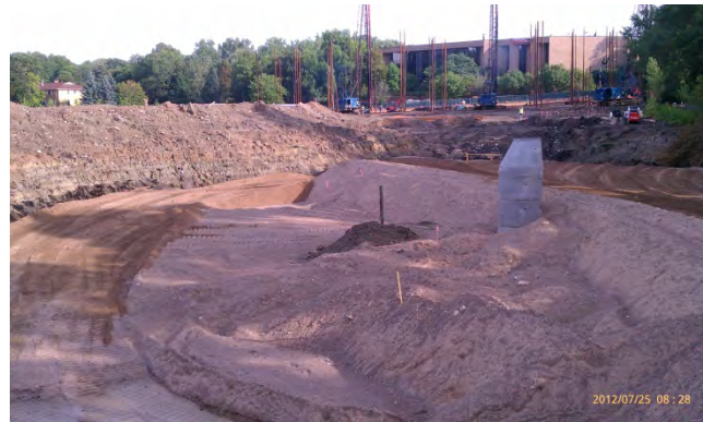
Imported clean sand fill in excavation for Engel Street infiltration basin (foreground). Steel pipe pile driving for Phase 1 building (background).
