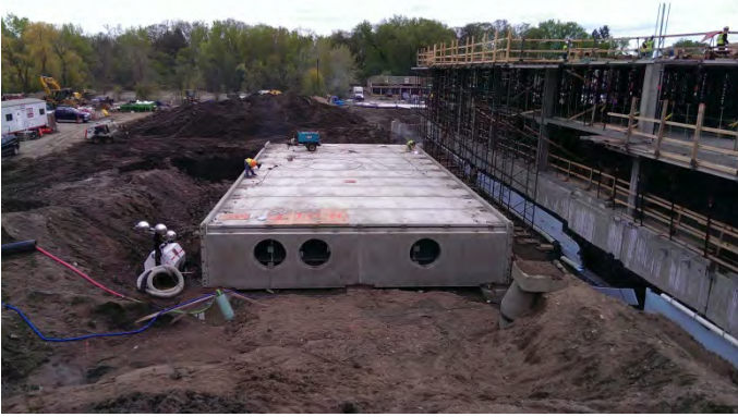
Looking south at Engel Street detention vault during construction. Three large openings are for connecting 48-inch perforated pipe network of adjacent infiltration basin.
