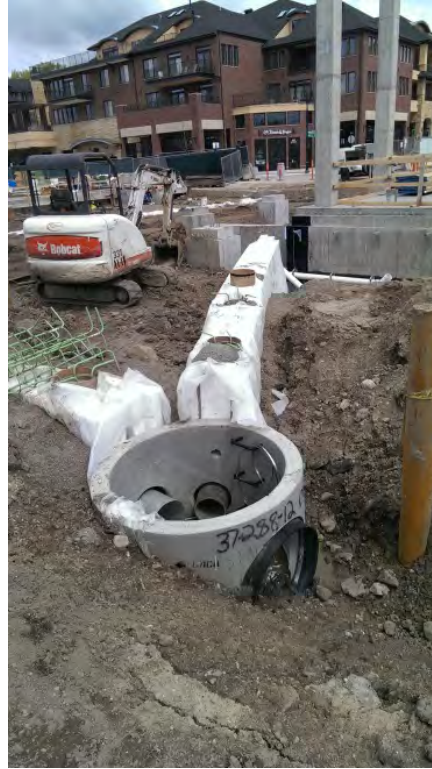
Storm sewer at The Promenade of Wayzata uses lightweight insulation "backfilled over pipes with poly sheeting "slip sheets" on sidewalls. Sonotubes centered over hanger connectors to be filled with reinforced concrete during subsequent post-tension slab pour.
