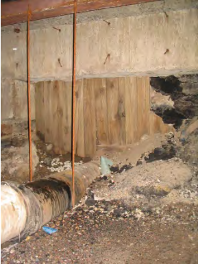
Roof pipe (white) connected to exterior storm sewer (black) – a flexible coupling between the two pipes is under stress from exterior settlement at the existing mall.
