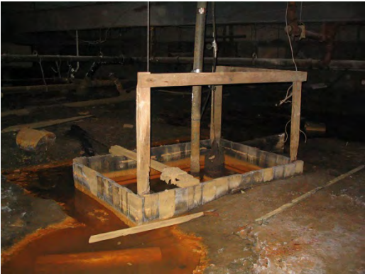
Makeshift sump pump to manage constant water in “crawl space” below existing mall.
