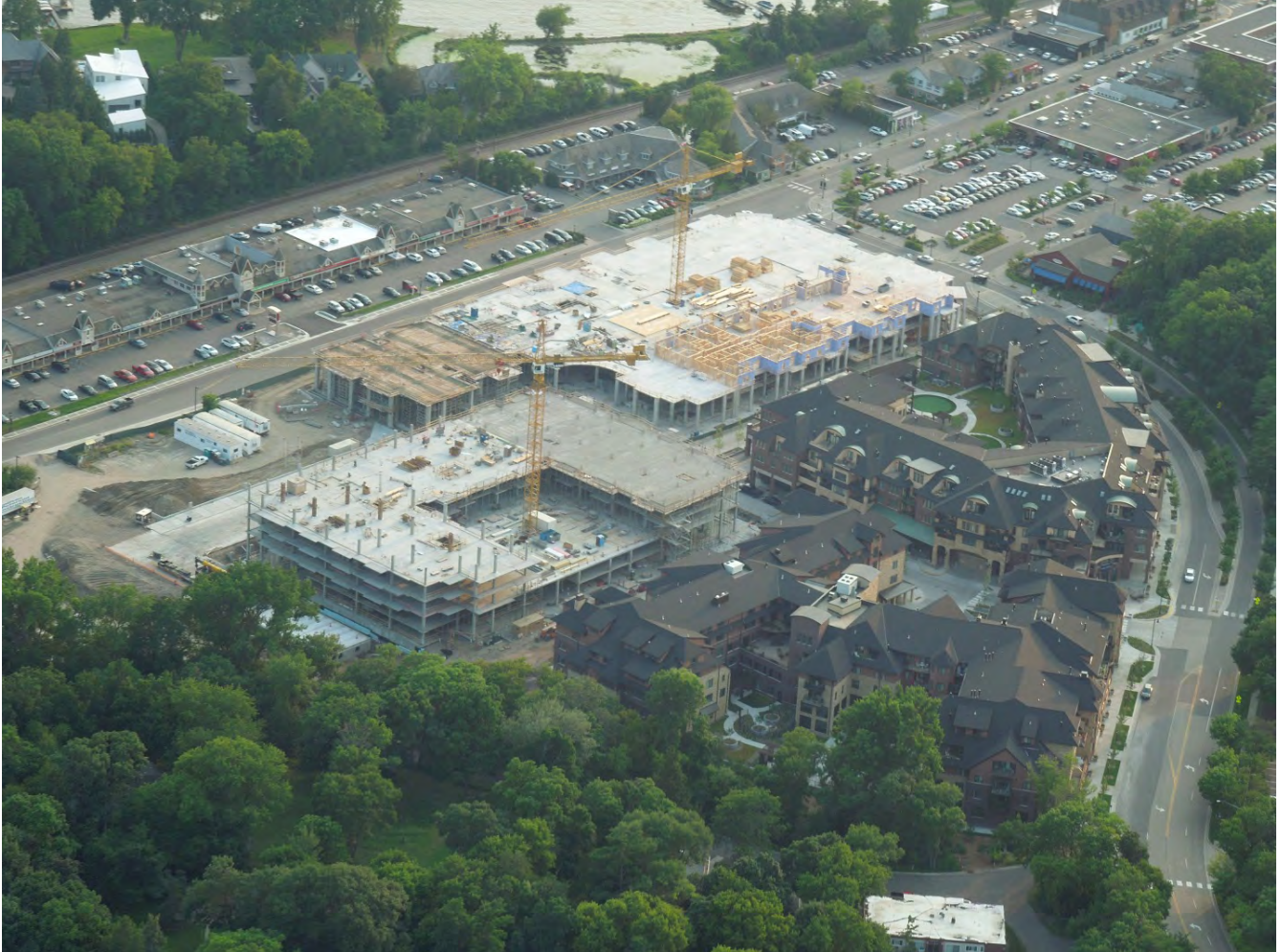
The new Promenade of Wayzata 14-acre mixed use redevelopment on the east edge of downtown Wayzata, Minnesota in mid Phase 2 construction (Phase 1 complete). Lake Minnetonka visible at top of photo. Photo courtesy of Brenda Chamberland, Aerial Solutions.
