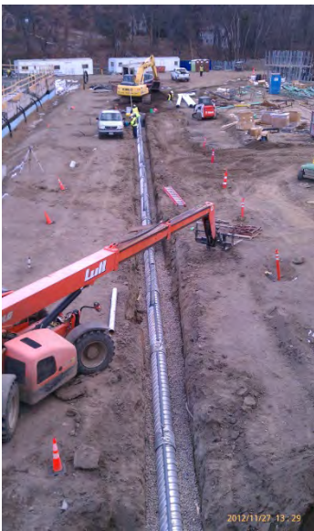
Unconventional storm pipe installation at The Promenade of Wayzata.
