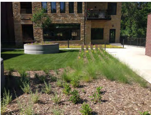
Lawn and planted area on The Terrace green roof of the Folkestone Terrace North (fka, North Block).
