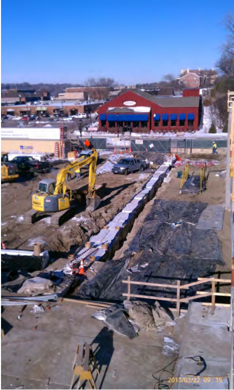
Storm sewer extending from Mill Street filtration basin. Lightweight insulation "backfilled" over pipes with poly sheeting "slip sheets" on sidewalls. Sonotubes centered over hanger connectors to be filled with reinforced concrete during subsequent post-tension slab pour at The Promenade of Wayzata.
