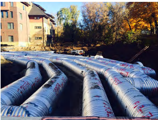
Perforated 48" corrugated metal pipe infiltration pipe installation at Engel Street infiltration basin. No alternative support for pipes is required since the soils on which the pipes bear are corrected inside the SCISZ. {SEE DRONE FLY-OVER OF THIS SYSTEM IN MID CONSTRUCTION @ www.youtube.com/watch?v=1iz_thP_1c&feature=youtu.be } Photo courtesy of Contech.
