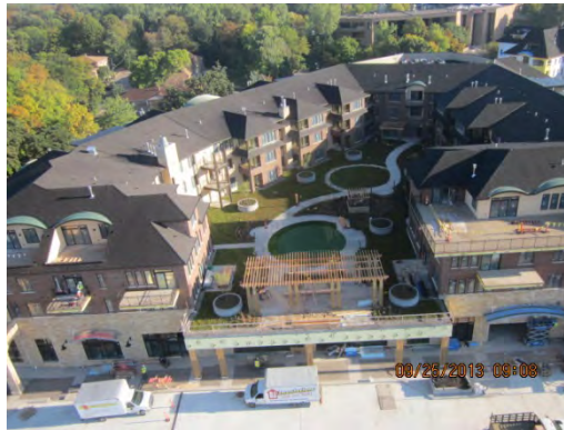
Recently completed green roof of the Folkestone Terrace West (fka, Superior Block). Photo courtesy of Adolfson & Peterson Construction.
