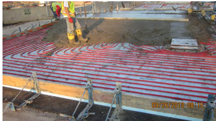
Concrete pour over hydronic snow-melt tubing around stormwater inlet grate at street intersection of The Promenade of Wayzata.
