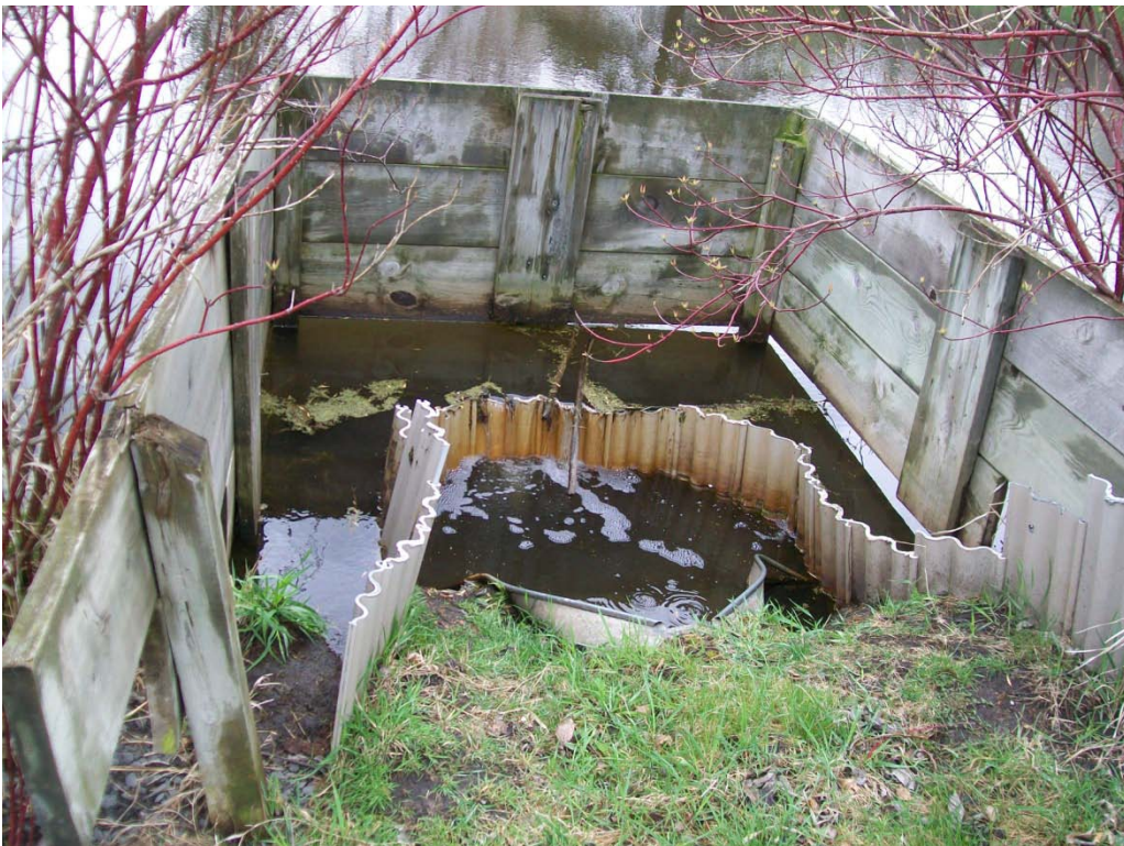
Photo 38: Outlet control structure located within residential pond south of subject wetland.
