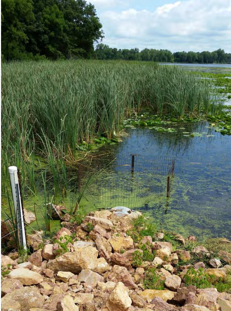
Figure 36. A photograph of the barrier in place at the Zumbra Lake outlet to Sunny Lake in the Carver Park Reserve. Lake levels were observed overtopping this barrier in August of 2016.
