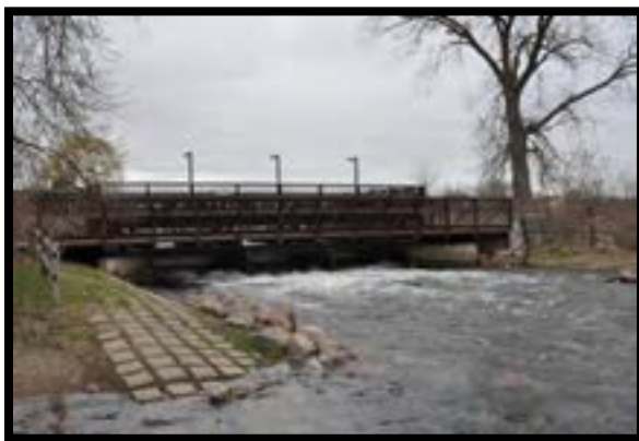
Grays Bay Dam May 1, 2014
