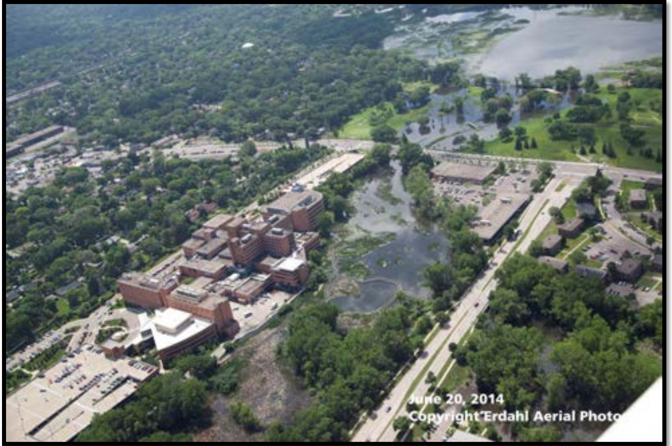
Flooding at Methodist Hospital and Meadowbrook Lake
