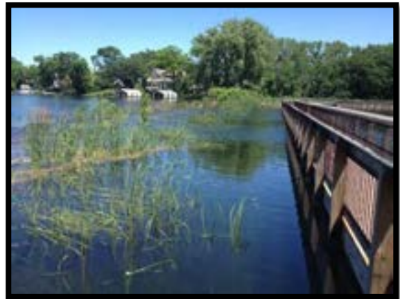
Emergency Spillway June 20, 2014
