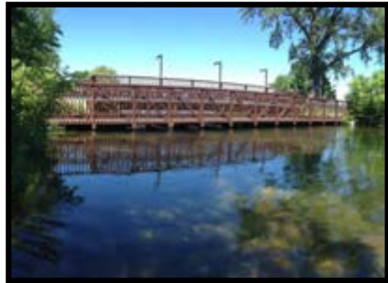
Grays Bay Dam June 20, 2014
