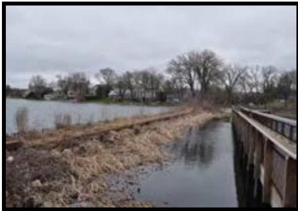
Emergency Spillway May 1, 2014
