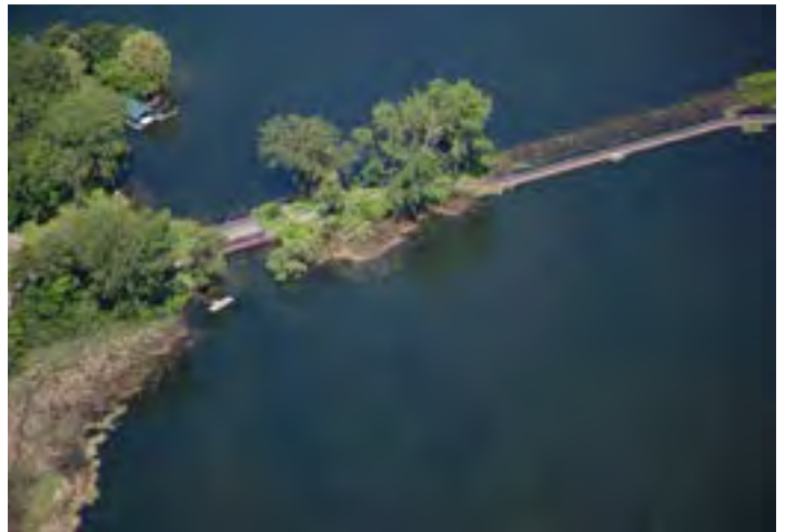
Gray's Bay Dam
