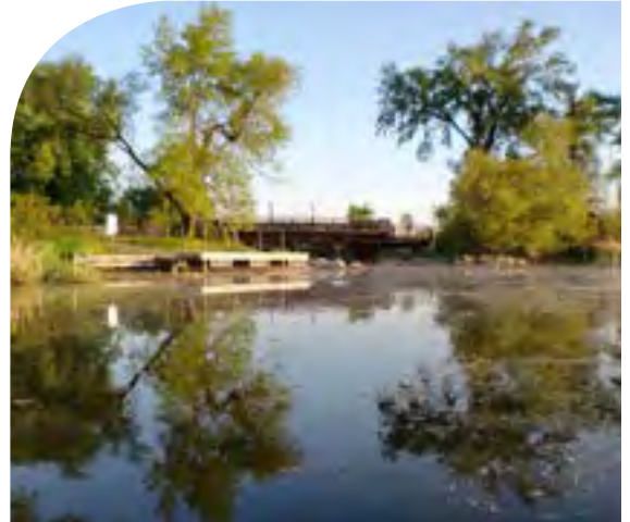
Grays Bay dam, Dale Antonson
