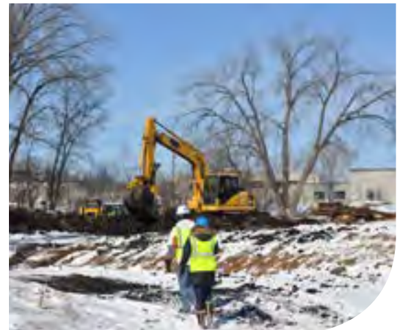
Staff inspecting a construction site
