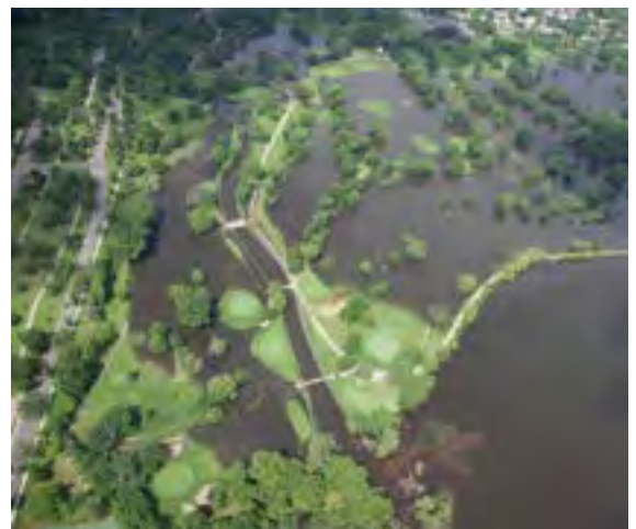
Lake Hiawatha during the 2014 flood, Erdahl Aerial Photos
