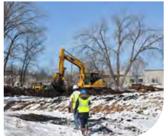
Staff inspecting a construction site
